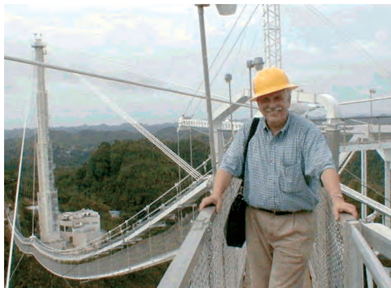
suspended Gregorian trusswork, 2001 (Inset: aerial view showing truss suspended 500 ft above the dish)
